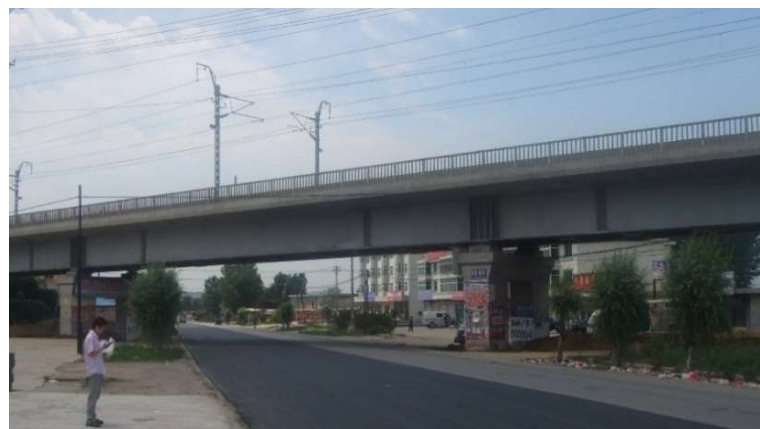
(32+40+32) m钢-混结合梁桥
